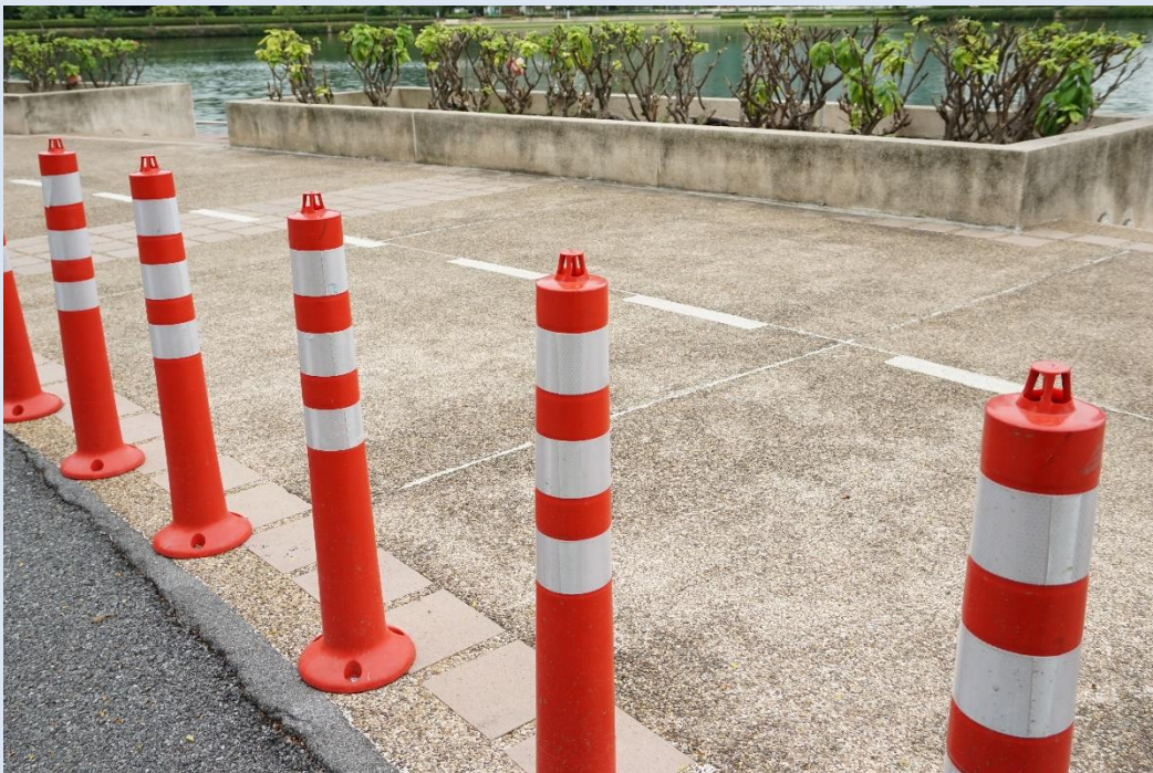
Figure 14. Flexible posts to separate cyclists from motorists
